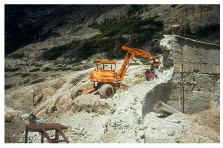
Figure 27. Schaeff Walking Excavator with hydraulic hammer was used in the deconstruction of Bluebird Dam to reduce concrete impacts on downstream greenback cutthroat trout populations (USSD 2015). (Photo credit Karpowicz et al. 2010).
