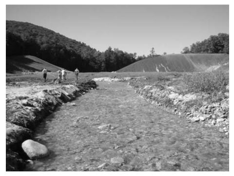
Figure 25. Conococheague Creek restored to its historic alignment with the breached Birch Run Dam downstream (USSD 2015) (Photo courtesy of Johnson et al. 2007, all rights reserved).
