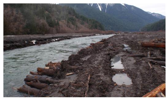
Figure 22. A pilot channel excavated through the Lake Mills delta and alder forest growing on the delta was cleared in preparation to remove Glines Canyon Dam near Port Angeles, Washington (USSD 2015) (Reclamation, December 2010).
