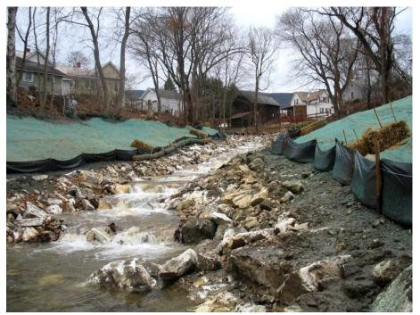
Figure 29. The restored step-pool system constructed in Hoxie Brook (USSD 2015) (Photo courtesy of Leone et al. 2010, all rights reserved)
