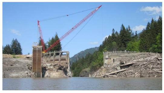
Figure 11. A large ringer crane was employed at Glines Canyon Dam, Washington in 2015 (Reclamation/Randle).
