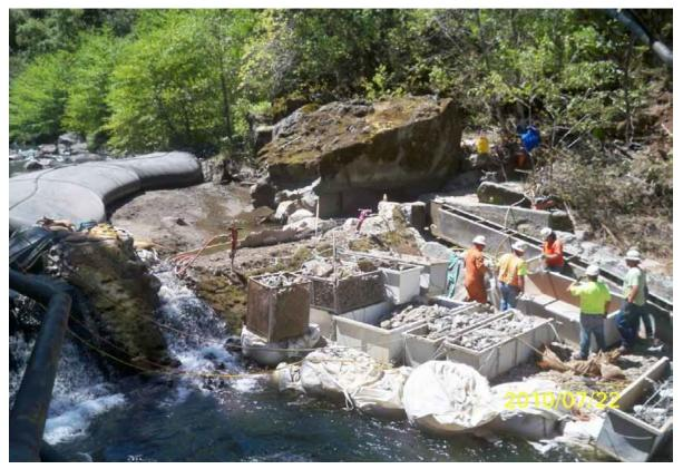
Figure 13. Temporary cofferdam and diversion pipeline designed and constructed to isolate the left end of Wildcat Dam on the North Fork of Battle Creek in California (Reclamation).
