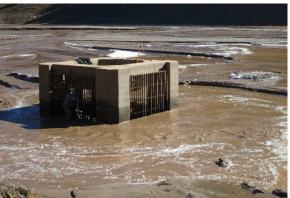
Figure 4. The outlet for Paonia Dam, near Paonia, Colorado, was constructed 21 m above the valley bottom in July 1961.
