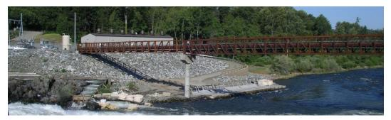
Figure 7. Pump station designed and constructed on the Rogue River in Oregon to replace gravity diversions from Savage Rapids Dam. A pipe bridge was constructed so water could be delivered to both sides of the river (USSD 2015) (Reclamation/Hepler).
