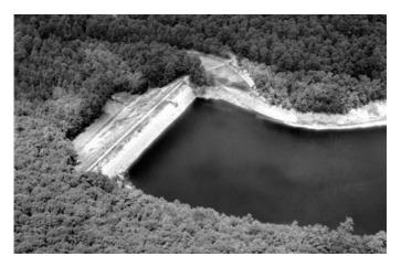
Figure 24. Birch Run Dam before breaching. The spillway can be seen on the right dam abutment (USSD 2015) (Photo courtesy of Johnson et al. 2007, all rights reserved).
