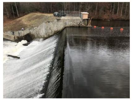
Figure 31. Repaired Rising Pond spillway and right embankment. (EPA 2020)
