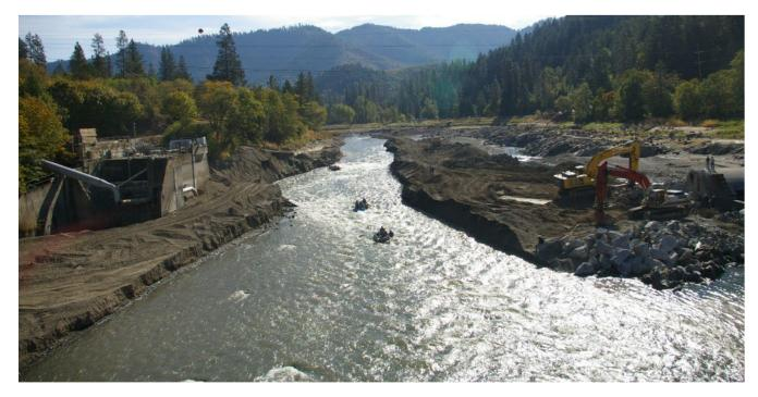
Figure 21. River erosion of reservoir sediments past Savage Rapids Dam near Grants Pass, Oregon, following dam removal (USSD 2015) (Reclamation/Bountry October 2009).
