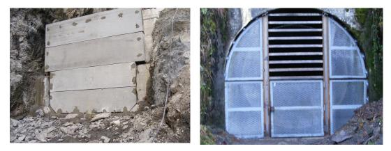
Figure 15. At Glines Canyon Dam, Washington, the upstream tunnel barrier (left) was blocked using precast concrete panels while the downstream tunnel barrier (right) was blocked using metal panels (USSD 2015) (Reclamation/Hepler).
