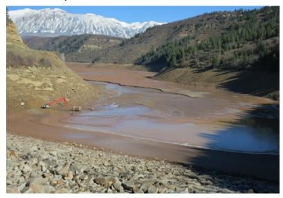
Figure 6. By 2014, reservoir sedimentation had filled 25 percent of the storage capacity and plugged the dam outlet at Paonia Reservoir in Colorado.
