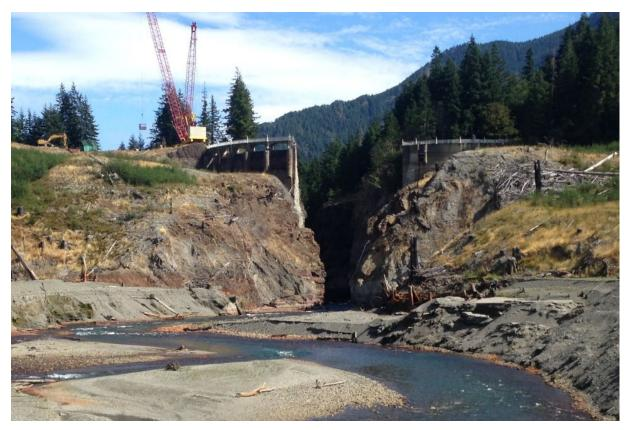
Figure 9. At Glines Canyon Dam, the left-side spillway gates and the right abutment thrust block were retained for a public overlook within Olympic National Park in Washington (Reclamation/Randle).
